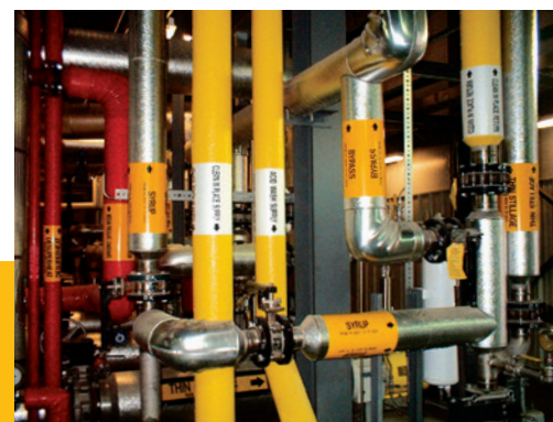
Typical marker installation
