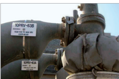
Installed control valve tags
