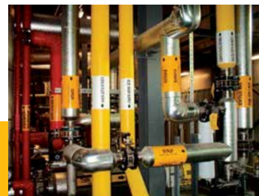
Typical marker installation
