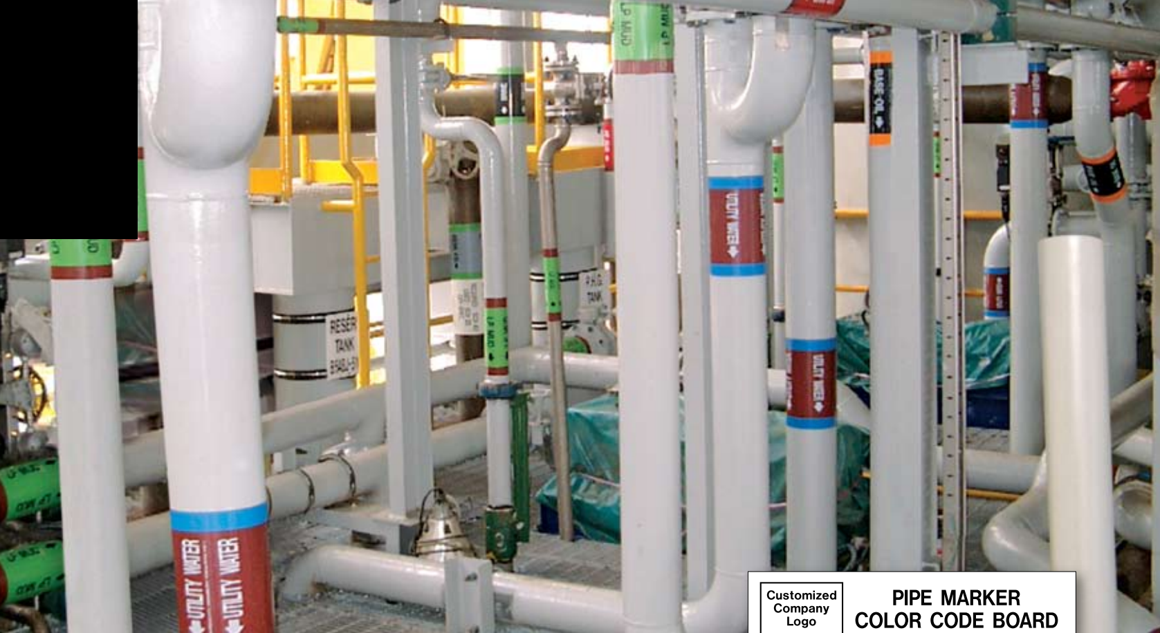
Typical pipe marker installation
